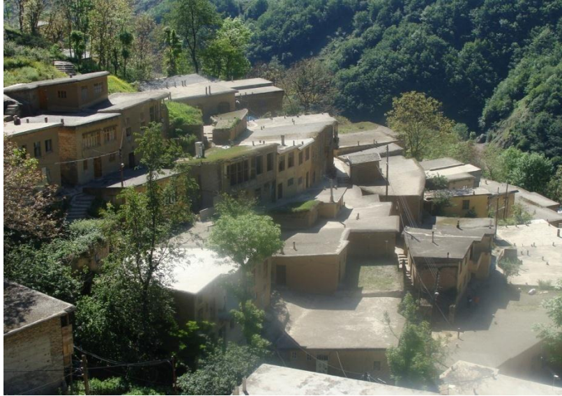
Figure (2): The architecture of Masoule village
